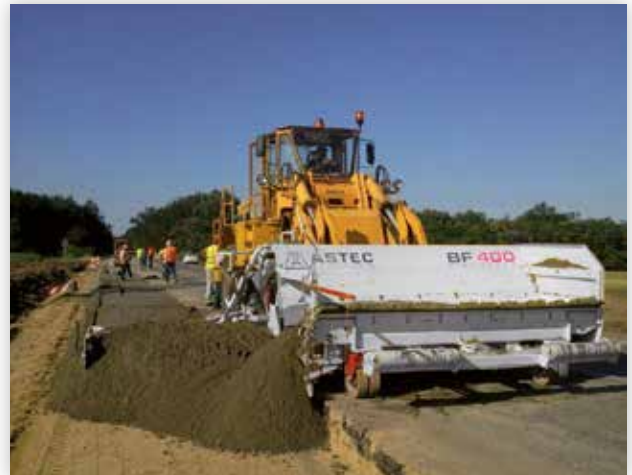
Road extension with 2 m working width
