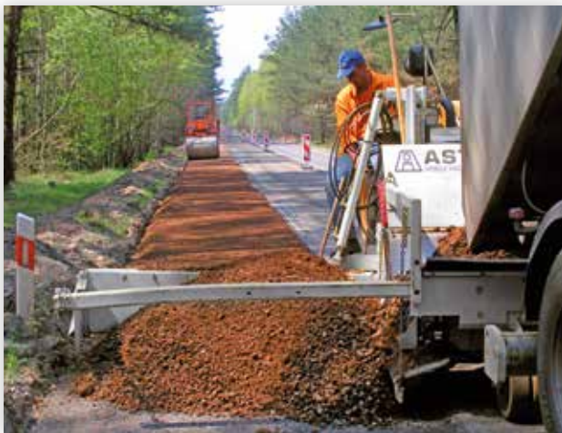
Road extension with 2 m working width – capacity for 400 to per hour
