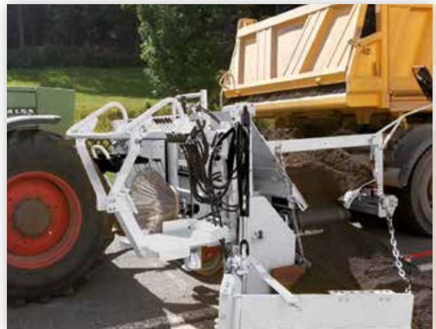
Excellent material flow on construction site
